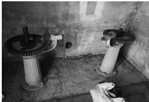
Cranks that Open and Close the Steel Doors inside the Dam
